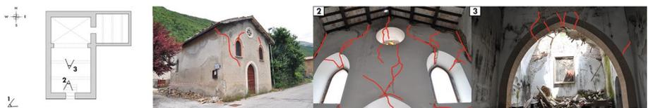
**Fig. 10** Damage survey in the church of Sant'Antonio in Ussita after the Central Italy Earthquakes of 2016
