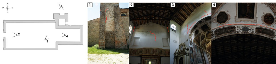
Fig. 7 Damage survey in the church of San Francesco in Montefortino after the Central Italy Earthquakes of 2016
