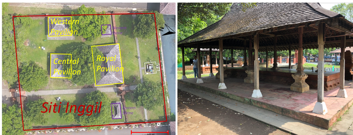
Figure 1. The area of Siti Inggil within the palace compound, which was documented in higher detail. To the left, an aerial view of the area with several main structures overlaid. To the right, the Royal Pavilion of the Siti Inggil compound. Note the characteristic tropical architecture in the form of double-tiered roofs and the absence of walls.
