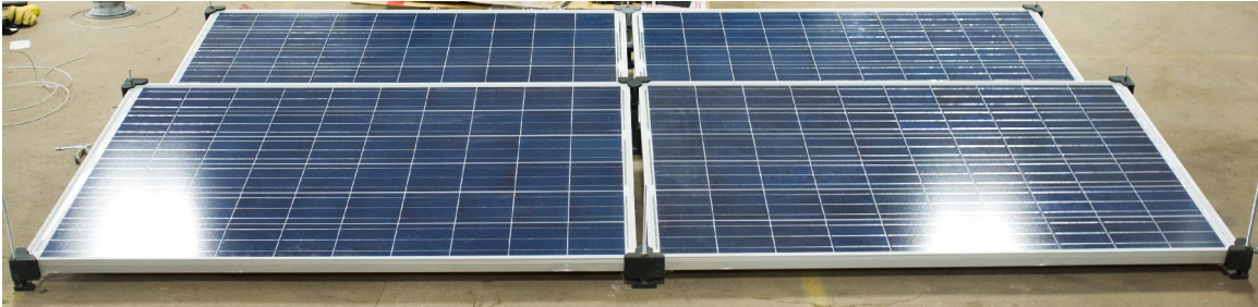
Figure 6: Assembly of 1kW X-wire racking system.
