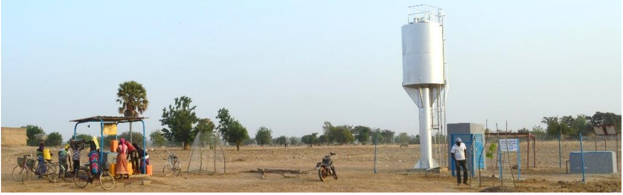
Figure 3 Overview of the PVWPS On the left: the fountain where the inhabitants collect water. On the right: the PV modules and the water tank surrounded by a wire netting
