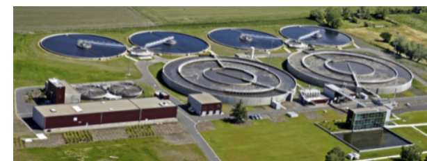
Urban waste water treatment plant
