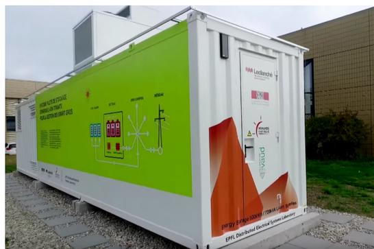
Fig. 1. The 720kVA/500 kWh grid-connected BESS installed at the Swiss Federal Institute of Technology of Lausanne (EPFL) used to validate the “dispatchable feeder” concept.
