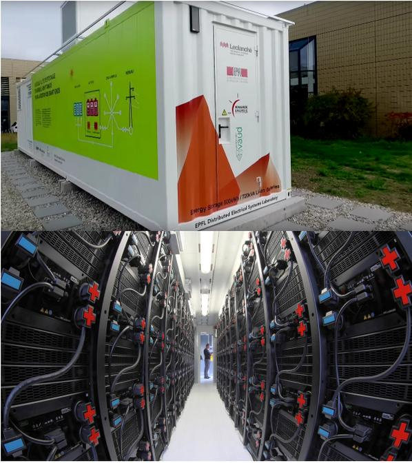
Fig. 8. An outside (top picture) and inside view (bottom picture) of the 720 kVA/500 kWh Lithium Titanate-based BESS used in this experimental work. The system, developed by Leclanché, includes a four-quadrant fully controllable DC/AC converter and a 0.3/20 kV step-up transformer. It is hosted in a temperature controlled container (picture of Alain Herzog, EPFL).
