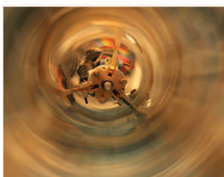
(B) Side view of the robot inside the pipe
