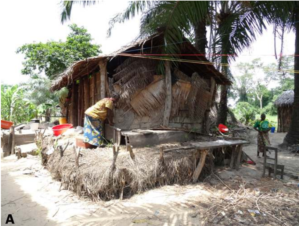
A: In the flood plain, people build earth mounds to protect their dwellings from seasonal flooding © M. COMPTOUR
