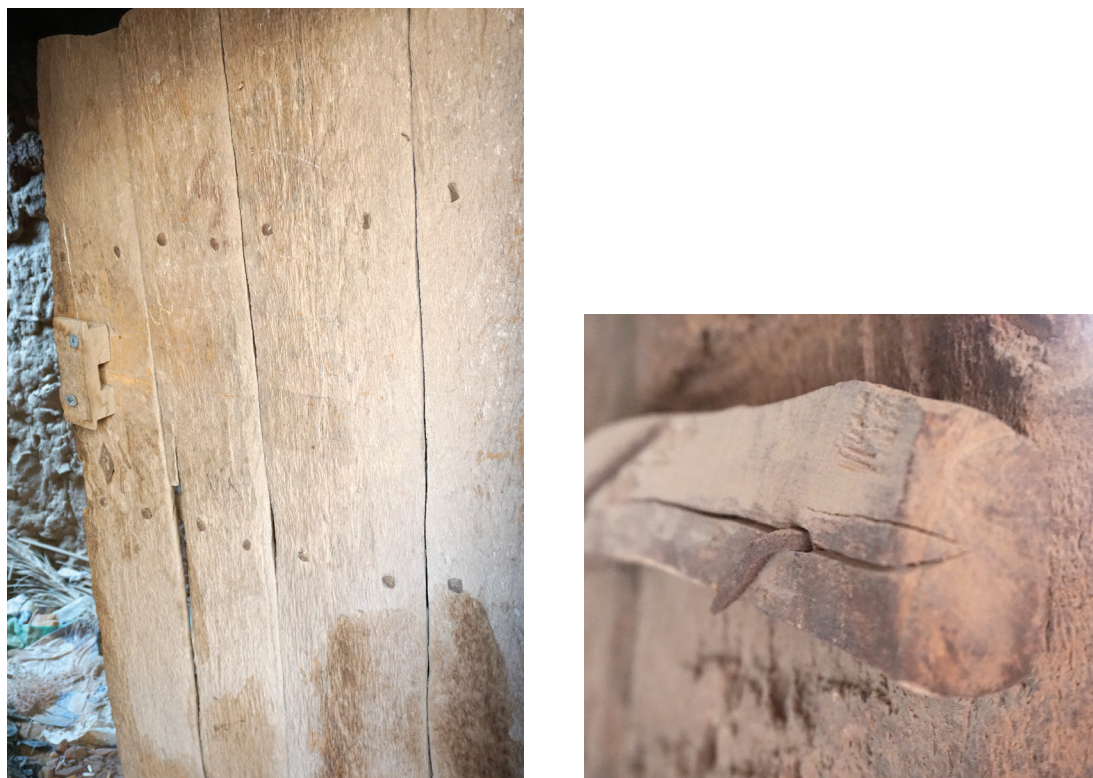
Fig. 2. Modern door in the old city of al-'Ulâ, made of several sections of date palm trunk (a) joined together with a transversal beam (Tamarix) and nails (b).
