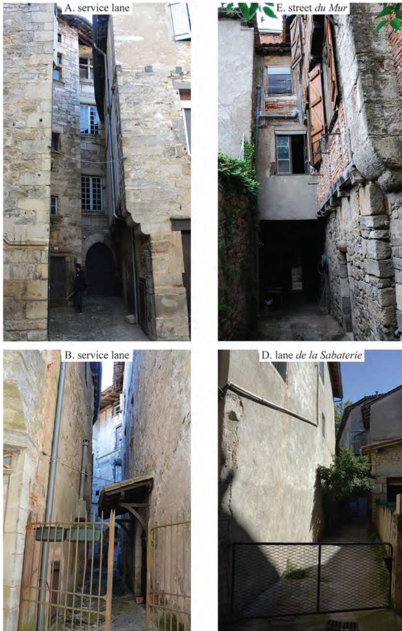
Fig. 13. Physical reality of streets and internal narrow streets of the block.
