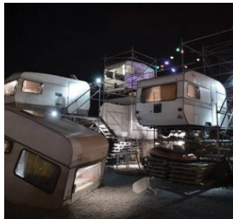
FIGURE 7 'Hameau de caravanes' - 'Hamlet of caravans'. The very first mini-housing facilities built on the campsite were 'Hameau de caravanes' (hamlet of caravans) - recycled caravans perched on scaffolds over two levels (Photograph by Yes We Camp! 2013).
