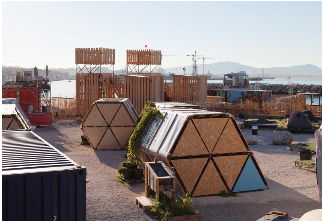
FIGURE 4 'Moissonneuses' - 'Combines' on the front and Perched Huts in the background. Dorms and small rooms built on scaffolds made out of wooden materials and recycled pallets and 'Les Cabanons perchés' (Perched huts) two-storey perched and shady platforms for tents built on scaffolds are among the flagship constructions of the camping. Designed by BC Architect & Studios and Michael Lefeber. (Photograph by Yes We Camp! 2013).
