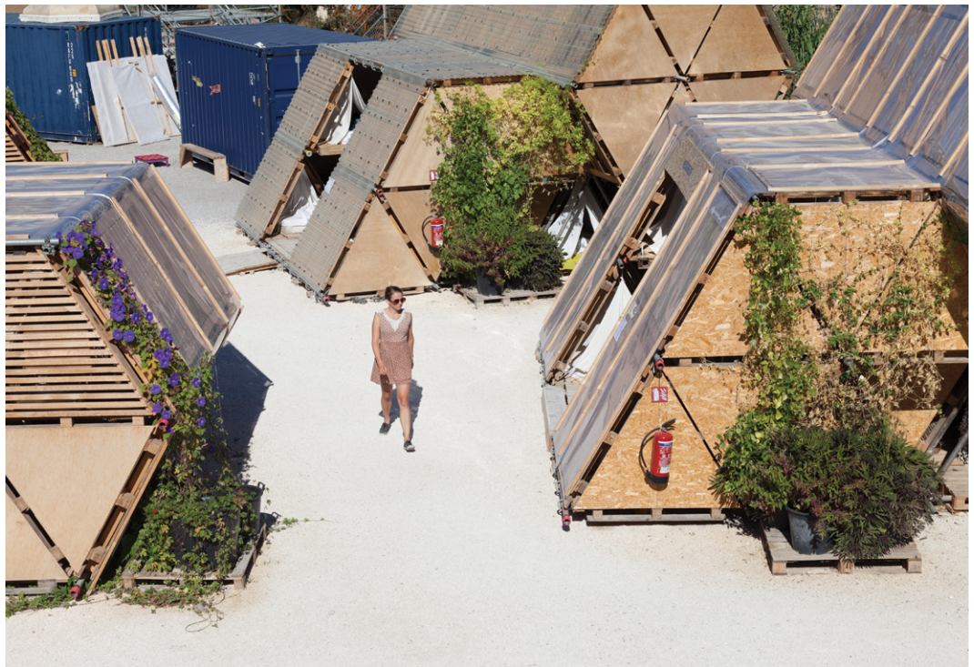
FIGURE 5 'Semeuses' - 'Sowers'. Dorms and small rooms built on scaffolds made out of wooden materials and recycled pallets. Designed by BC Architect & Studios and Michael Lefeber (Photograph by Yes We Camp! 2013).
