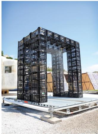
**FIGURE 14** Passage au frais. In addition to the main mini-housing and functional constructions, numerous landscape constructions and 'bounty spaces' were created. One is 'Passage au frais' (Passage into the fresh) – a system of water spray constructed out of plastic boxes (Photograph by Yes We Camp! 2013).
