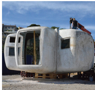
FIGURE 8 Bubble house. Designed in the sixties by architect Jean Benjamin Maneval, the habitat is composed of six plastic shells. It was first used in the campsite Elf Aquitaine and then recovered by a group of artists and performers. An example of architectural utopias of pop art, Bubble house was one of the emblematic habitats of the campsite (Photograph by Yes We Camp! 2013).
