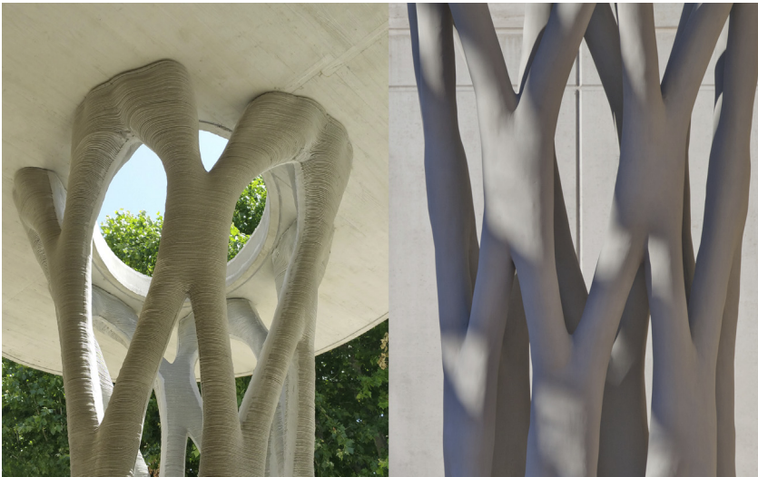
Figure 3.8 Before (left) and after (right, photo by Lisa Ricciotti) surface smoothing obtained through manual coating.
