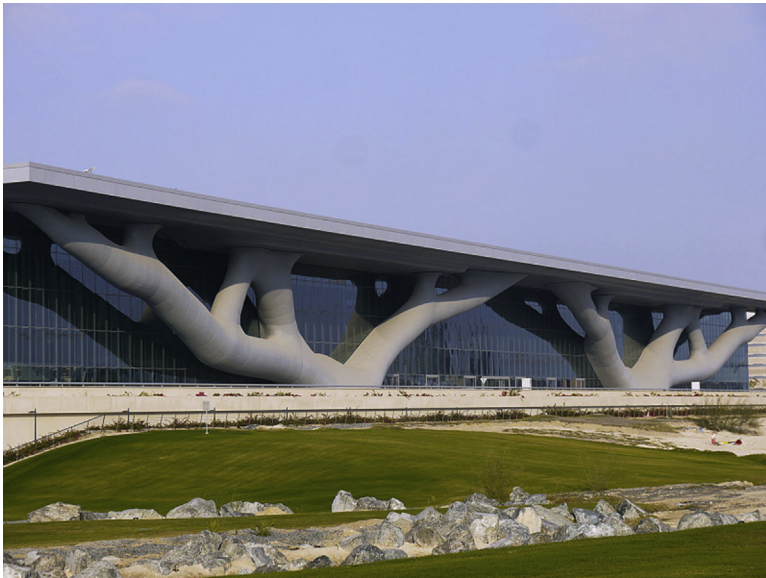
Figure 3.9 Doha Convention Center, with truss-shaped pillars.
