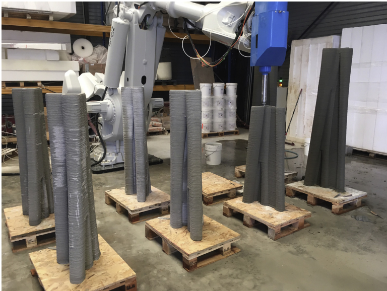
Figure 3.13 Concrete formwork 3D printing for the 4 pillars (2 parts per pillar).
