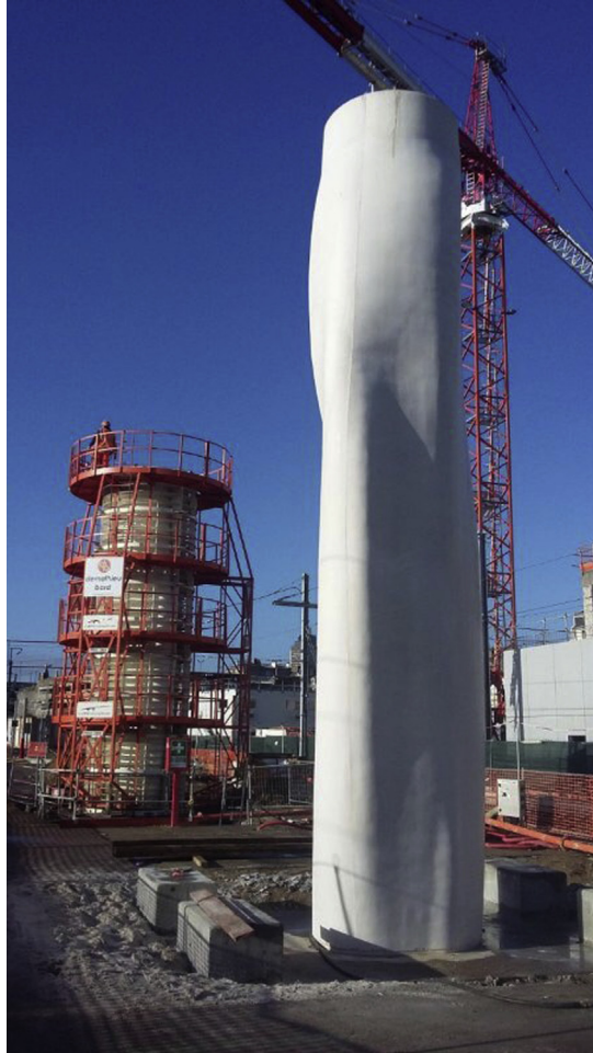
Figure 3.11 Example of semistandard shaped pillar on the construction site of the new train station of Nantes, France.
