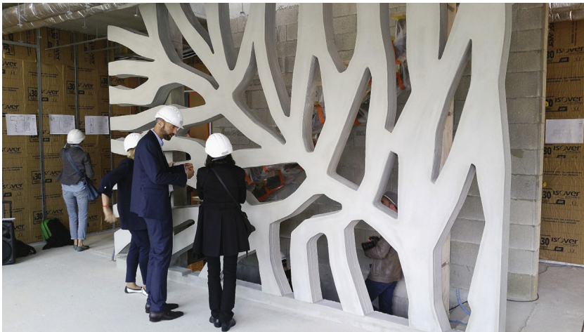
Figure 3.16 Interior wall made of the 3D-printed concrete formwork filled with cast concrete after finishing.
