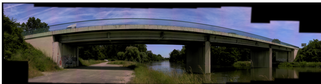
Figure 1. Example of a panoramic image captured with Trimble SX10 on a bridge using the primary camera and an overlap of 20% between individual pictures.
