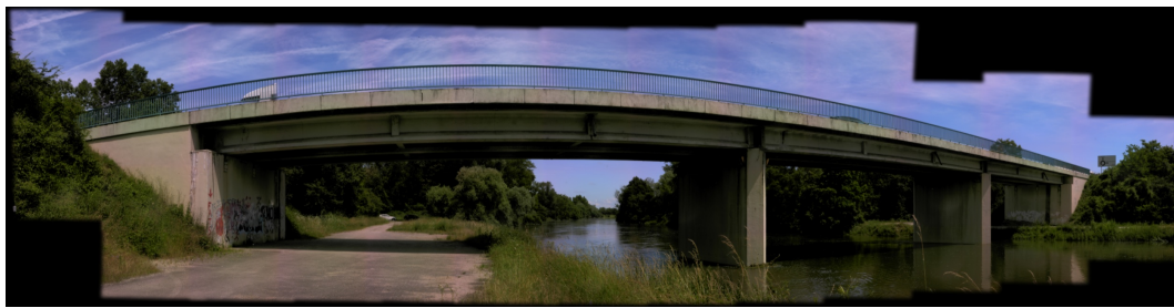
Figure 1. Example of a panoramic image captured with Trimble SX10 on a bridge using the primary camera and an overlap of 20% between individual pictures.
