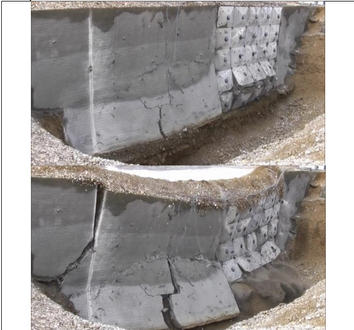
Figure 11. Collapse mode of two nail walls under explosion
