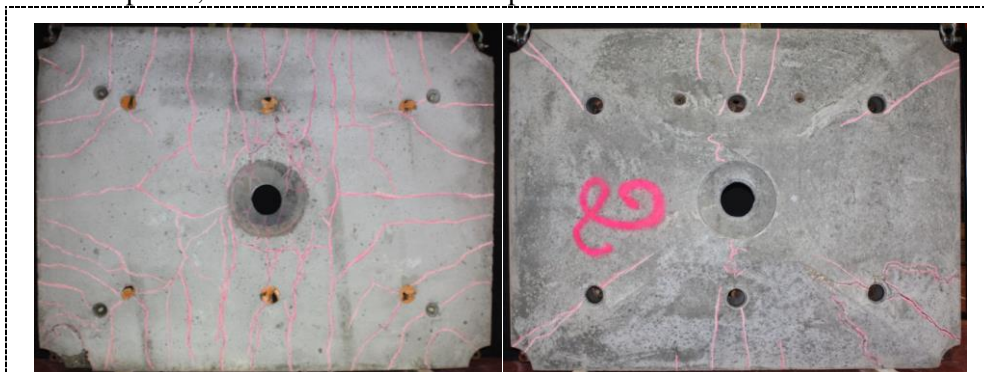
Figure 5. Failure modes of specimen 1: bottom face and top face
