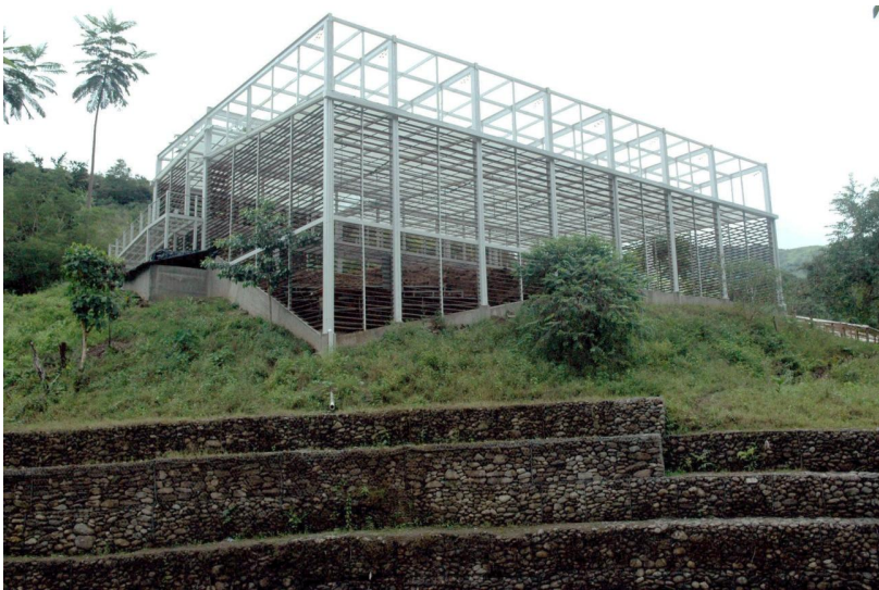
Figure 3 Interpretative center structure protects ancient architecture.
