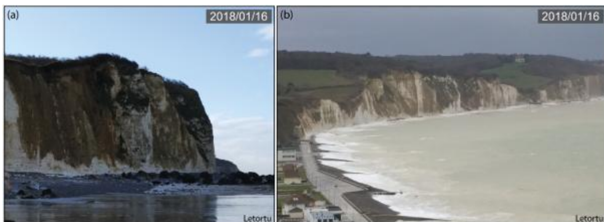
533 534 Fig. 11: Marine action visible after a stormy period (December 2017-January 2018) in 535 Varengeville-sur-Mer (a) with bleached cliff foot (b) and the removal of falls by dissolution 536 into the sea.
