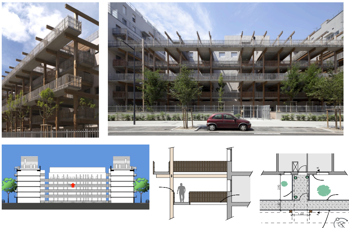
Figure 5b: The external corridor of the residential building in Caserne de Bonne – Grenoble, France. Urban section and architectural drawings representing the corridor and the balcony. Caserne de Bonne - Grenoble, France. Designed by Edouard François. (Above)
