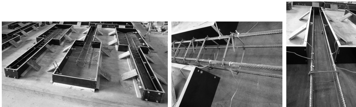
Figure 1. UHPFRC specimens: geometry and pictures of formwork and reinforcement before casting
