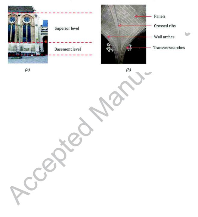
Figure 3. Different masonries in place in the monument: (a) elevation wall, (b) ribbed-vault
