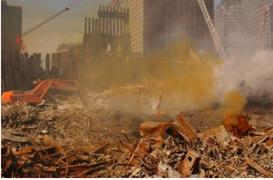
Figure 21: Some orange fumes observed at Ground Zero, from [63]
