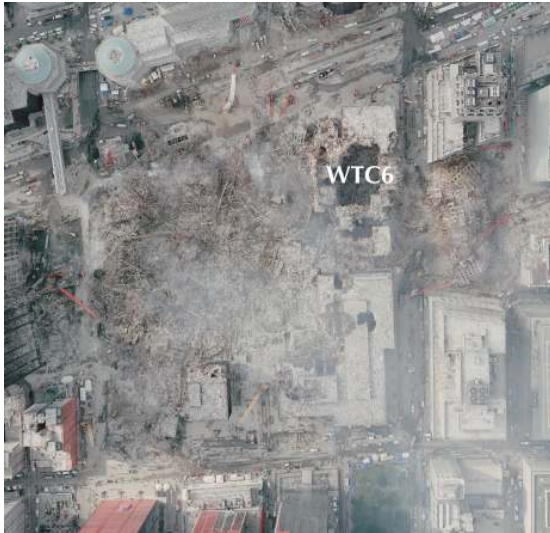
Figure 19: On this aerial photograph of World Trade Center, WTC6 building exhibits very large and deep holes (cropped from [55]).
