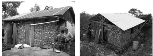
Figure 1: Rural Haitian house: (a) Traditional “Kay peyi” (b) Built for a reconstruction project
