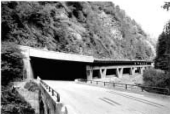
Figure 1. Les Essariaux Rock-shed
