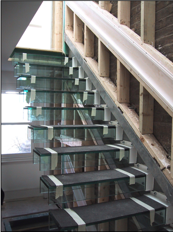
Fig. 2: Global structural system of glass stair (during construction)
