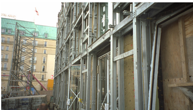
Fig. 5: Steel-girder construction of the façade
