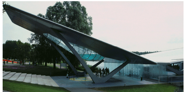
Figure 5: Glass pond of the Municipal Pavilion
