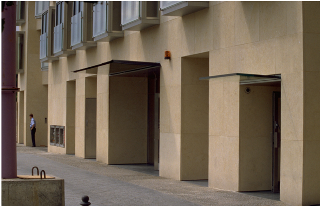
Fig. 16: Glass canopies at the building side facing Behrenstrasse
