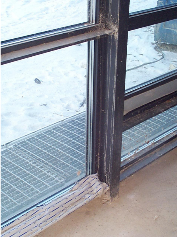
Fig 8: Double-skin structure connected to an I-section column
