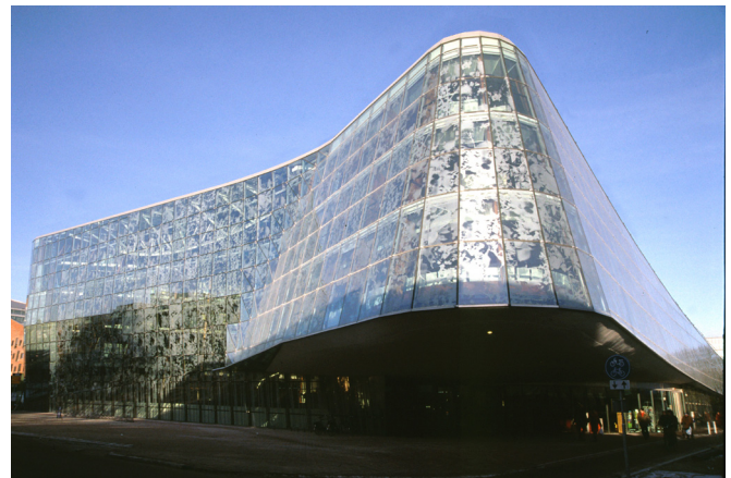
Figure 8: Exterior of the Town Hall with its triangulated and printed glass panels
