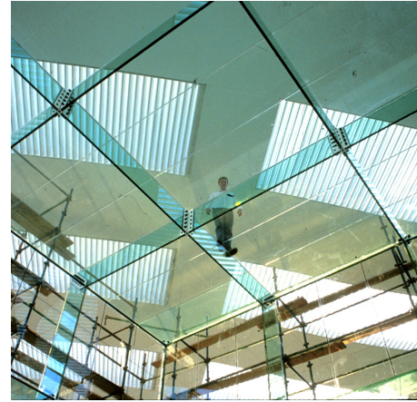
Fig 10: Detail of roof construction
