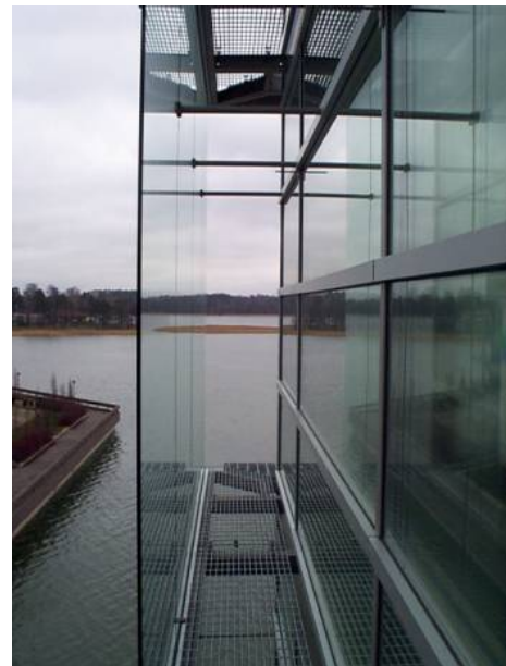
Fig 1: Cantilever beams as a supporting structure
