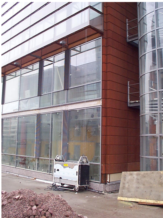
Fig 10: The service cage for the maintenance of the intermediate space.
