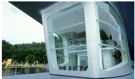
Figure 6: Cold deformed laminated glass panels
