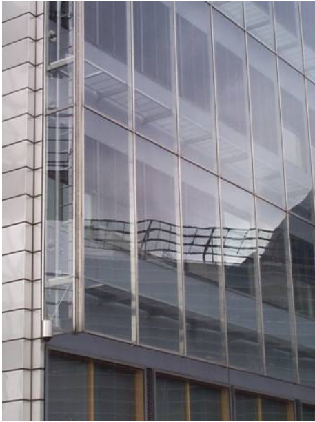
Fig 3: Vertical frames as a supporting structure
