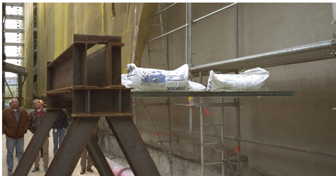
Fig. 9: Mockup for the impact tests at the construction site
