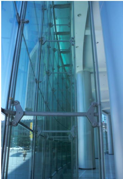
Fig 5: Vertical glass panels brace facade
