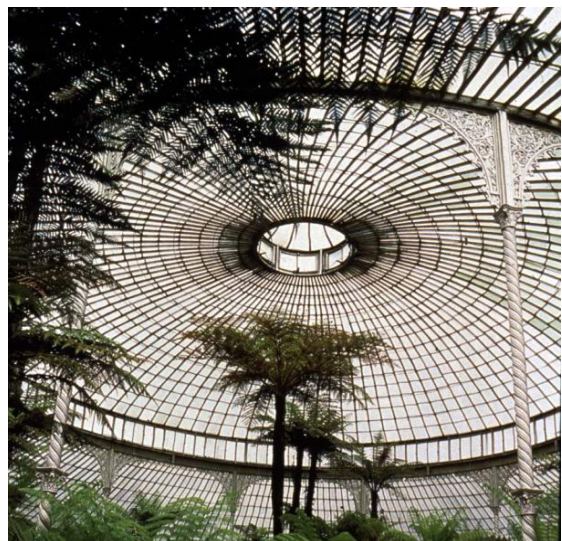
Fig.1 Kibbles Palace in Glasgow (1873). Note the slight out-of-plane curvature of the vertical iron arches on the right photo. This indicates the bracing action of the glass panels.
