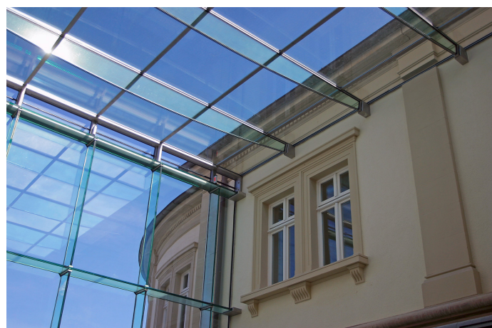
Fig. 4 Interior view of the roof structure
