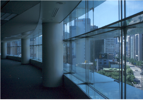
Fig 5: Horizontal glass beams span 12m
