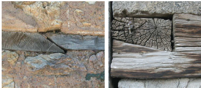
Figure 3: a) a chamfered joint in Vevçani (Macedonia) and b) a dovetail joint in Erzurum (Turkey) (Credit: Hofmann)
