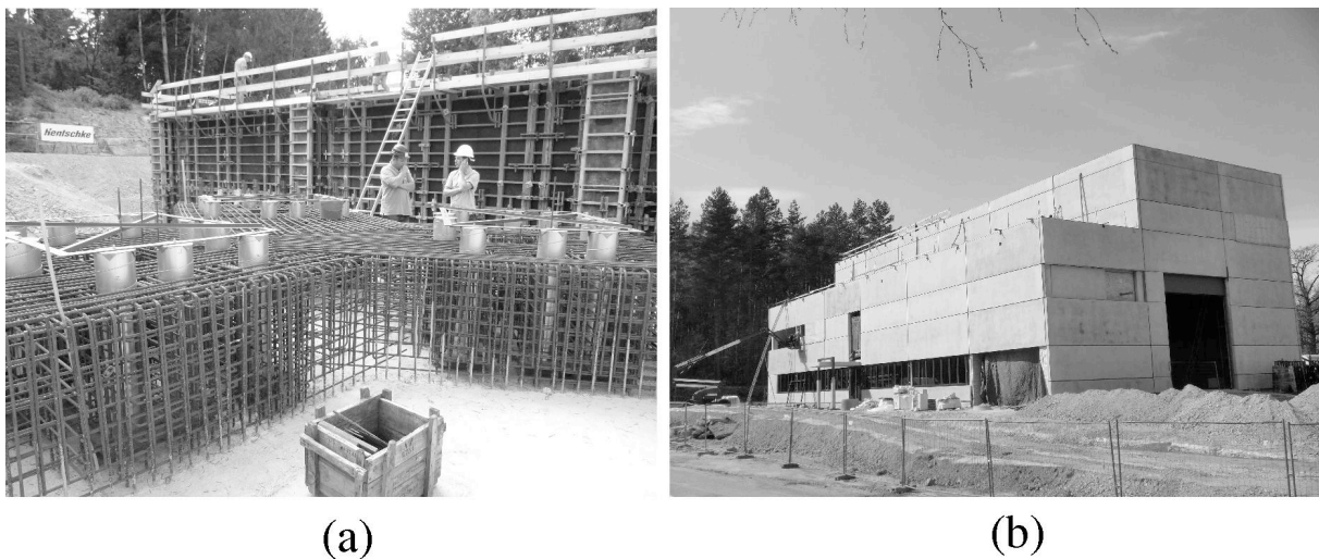
Figure 3: The DRESHDYN building: (a) Construction of the three feet of the precession experiment. (b) Present status of the shell construction (as of April 7, 2014).
