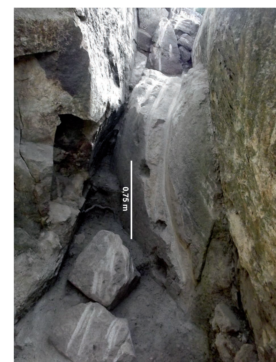
Notches in the wall below the stope
