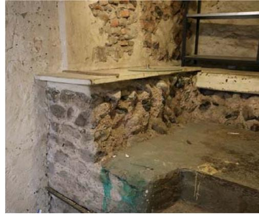
FIGURE 49 – 2 PLACE DE GORDES, SOUS SOL – PAREMENT DE L'ENCEINTE
