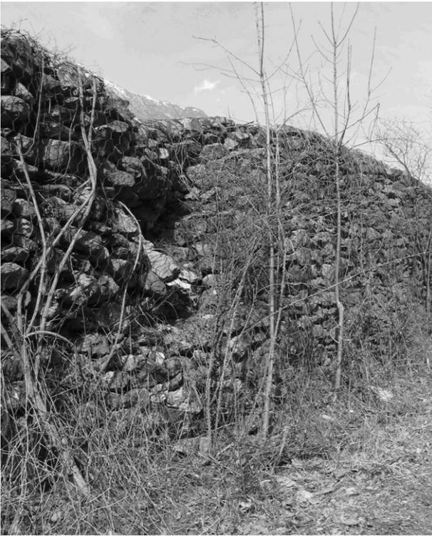
**Fig. 4.** This 3-m-tall gabion embankment was cleared by a block after an impact more than 1 m below its crest (Ste Marie de Cuines (73), France).
