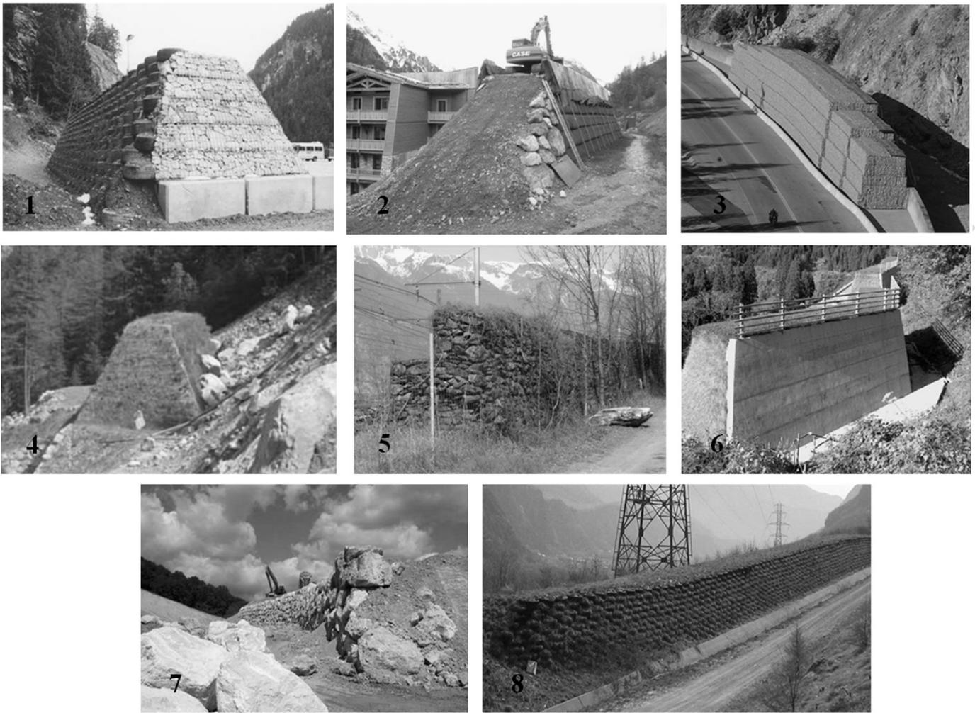
Fig. 1. Illustration of the variety of rockfall protection embankments (1: Coulon and Bruhier, 2006; 2: Lorentz et al., 2010; 3: Simmons et al., 2009; 4: Ronco et al., 2010; 5: author's collection; 6: Willye, 2003; 7 and 8: author's collection).
