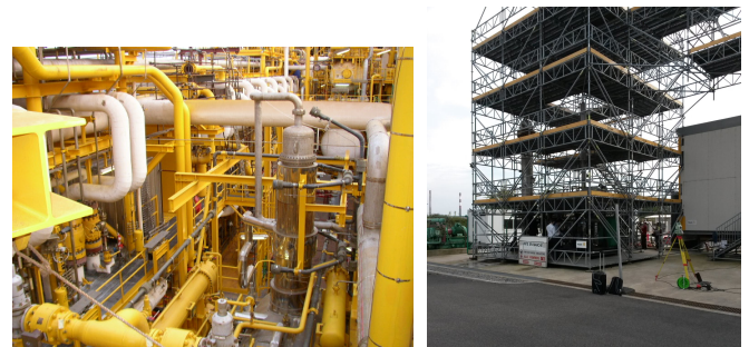
(a) Floating production storage and of- (b) ARGOS challenge test site floating boat. ©Serge RUPERT Total (UMAD) S.A.
