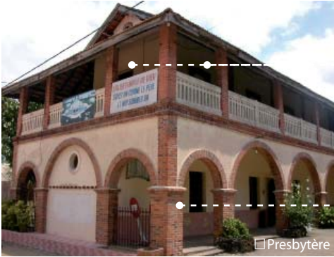
GALERIES (matériau, structure)
