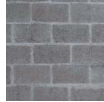
Mur brut parpaing ciment
