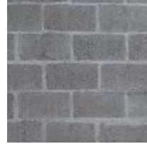
Mur brut parpaing ciment
