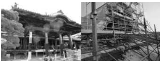
(a) Before demolition work (b) Demolition of roof frame
