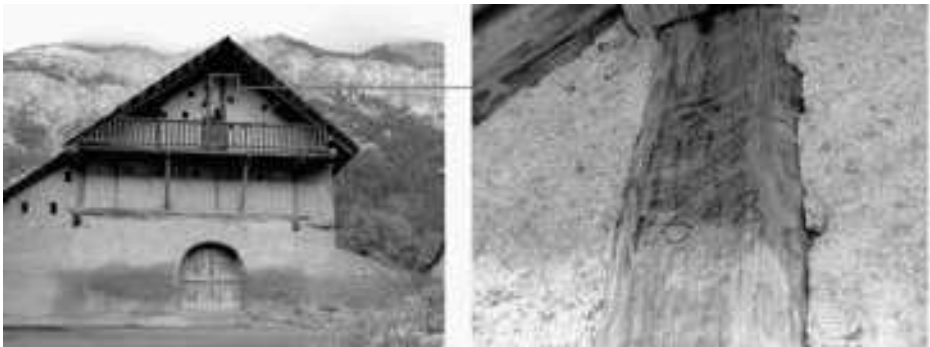
Fig. 2: Farmhouse, Val-des-Prés (05). Dating inscription details [IHS / 1648], on the western roof truss of the framework (photographs L. Shindo)
