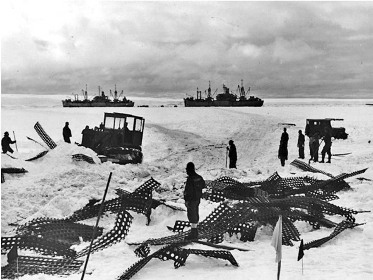
Figure 8.2. A bulldozer preparing a path during Operation Highjump to lay Marston matting and facilitate unloading of ships. Photo: US Navy, no copyright.
