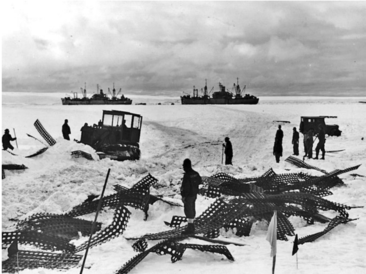
Figure 8.2. A bulldozer preparing a path during Operation Highjump to lay Marston matting and facilitate unloading of ships. Photo: US Navy, no copyright.
