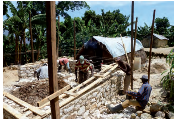
Above: horizontal wooden wall ties arranged at a 65 cm intervals
