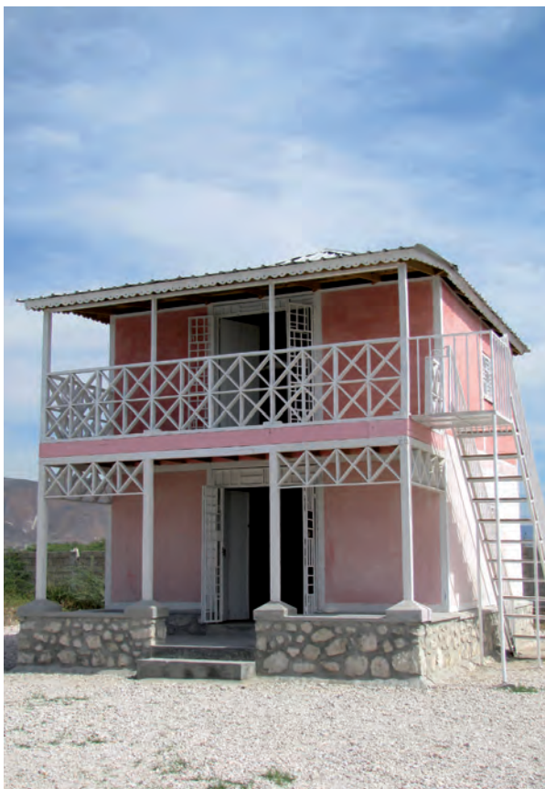
Below: two-storey building, business incubator, Corail Croix des Bouquets
