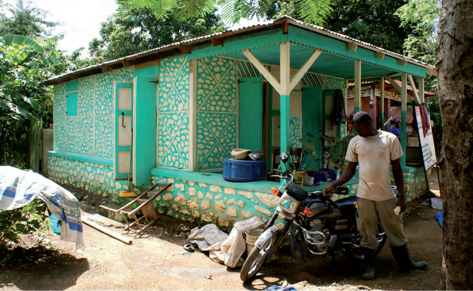
Above and left page: beneficiaries choose paint colours. The care they take to decorate the walls of their homes shows their pride
