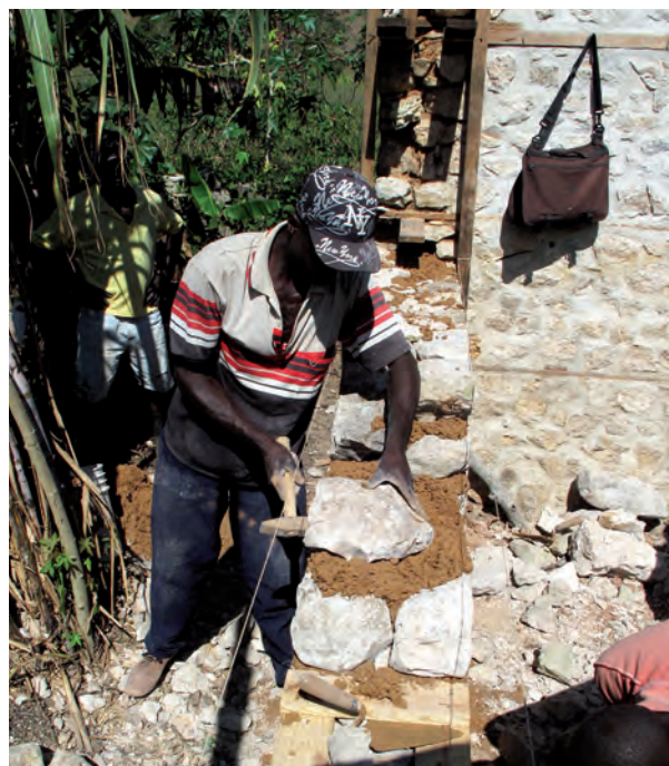
Below: stone and earth mortar masonry
