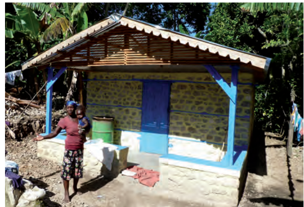
Below and left: different stone masonry houses
