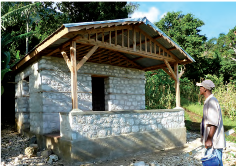
Above: stone and earth mortar masonry
