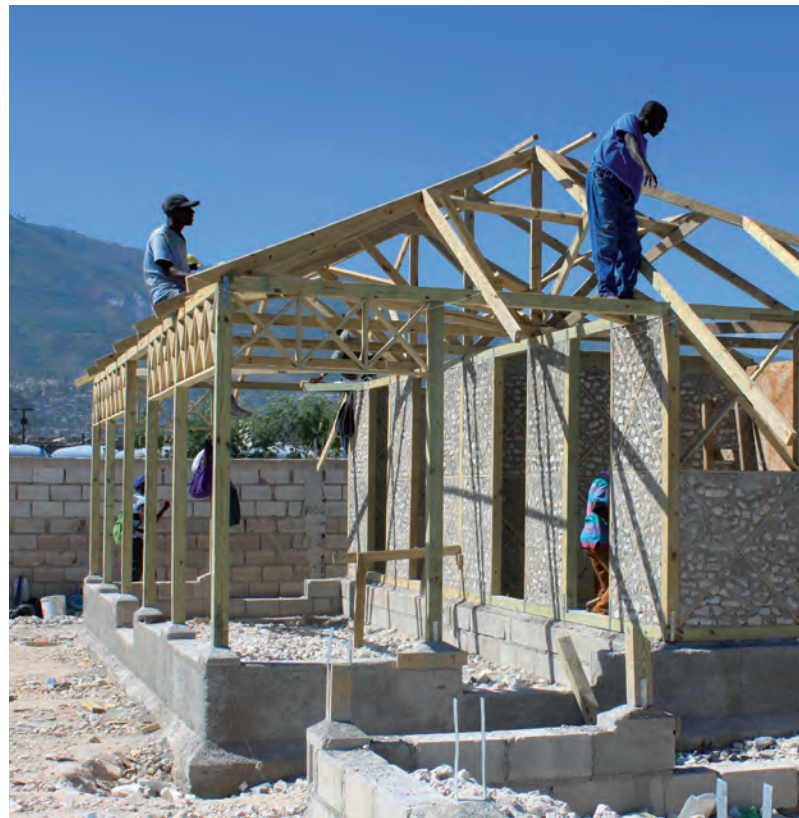
Wood frame wall panels filled with masonry debris
