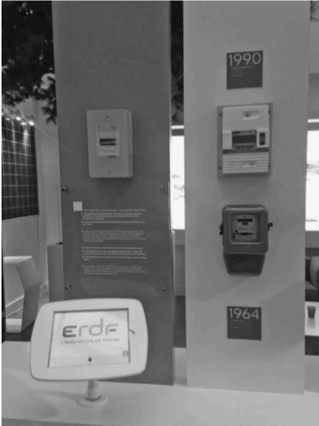
FIGURE 13.3 Electronic meters, introduced into homes in 1990 (right, at the top). We can also see one smart meter Linky (left). From 'The saga of the meter', electric meters in the exhibition showroom of the French electric distributor Enedis in Paris. Personal photograph.
