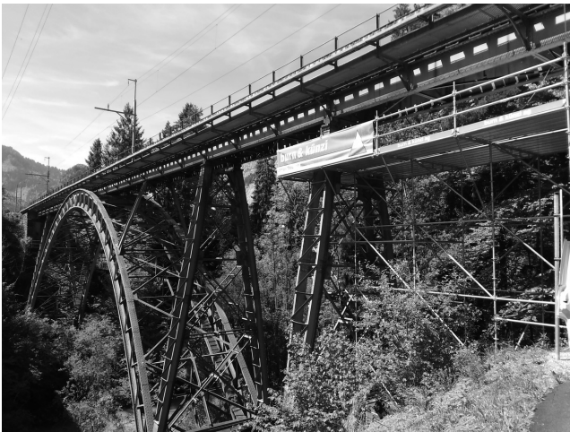
Figure 1 The railway bridge with the scaffolding for installation of monitoring.
