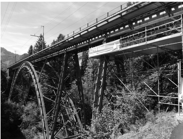
Figure 1 The railway bridge with the scaffolding for installation of monitoring.
