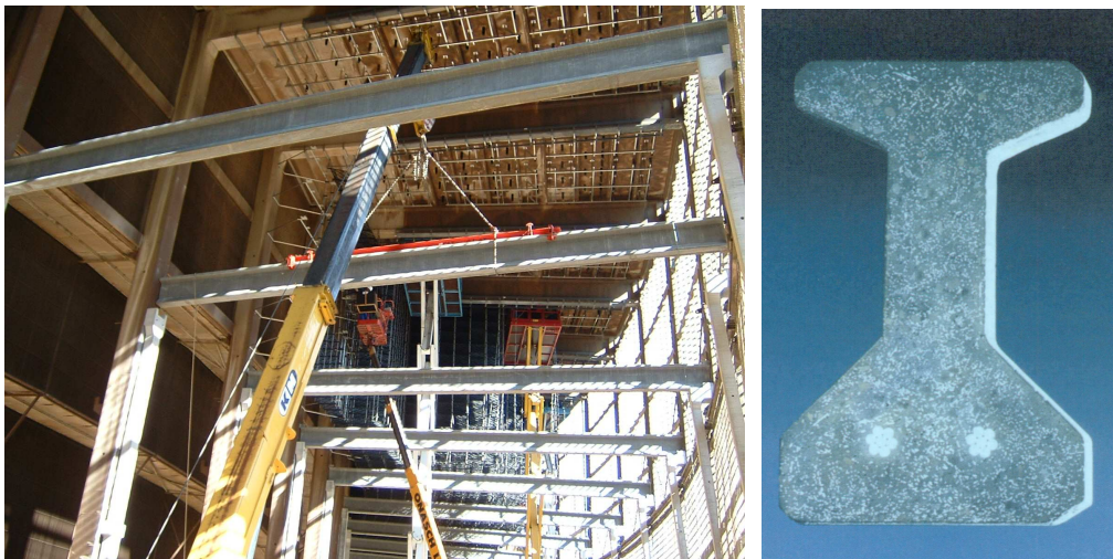
Figure 3: UHPFRC beams for thermal exchange devices in Cattenom NPP cooling tower [3]
