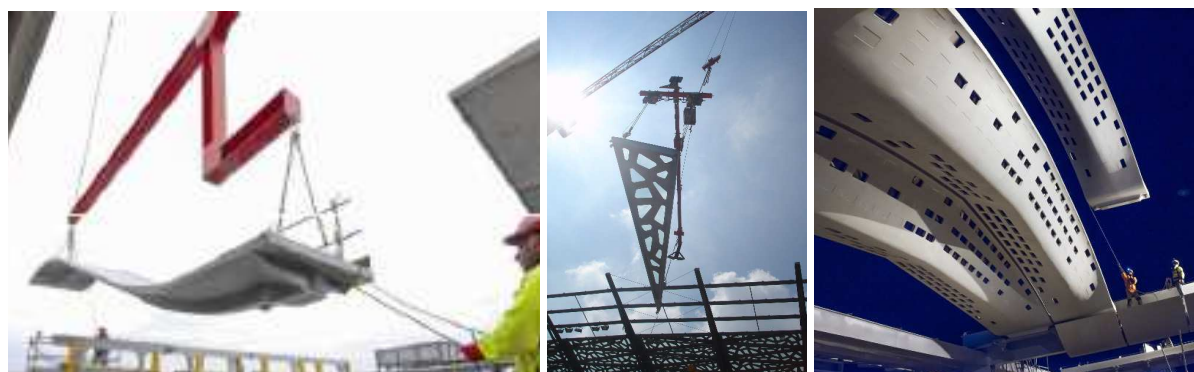
Figure 18: Typical handling operations of large and thin UHPFRC elements [34, 18, 35].
