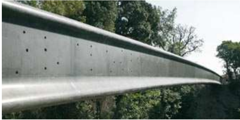
Figure 6: Passerelle des Anges, post-tensioned braced lateral beams, 1/38 slenderness [10]
