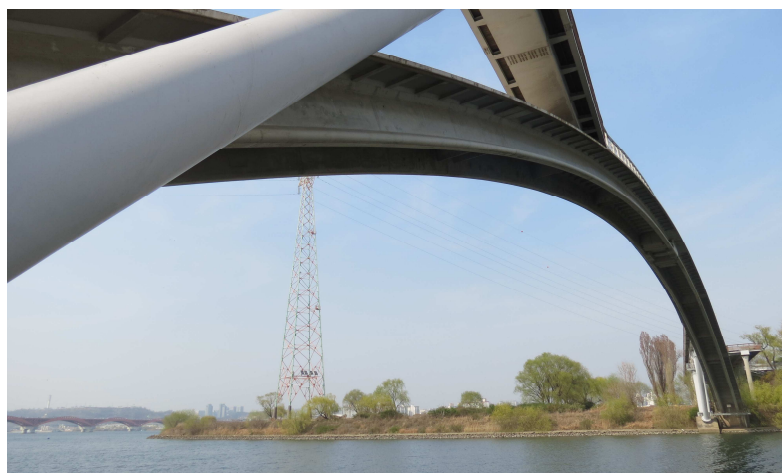
Figure 5: Pi-shaped cross-section of the UHPFRC arch Seonyu footbridge in Seoul.
