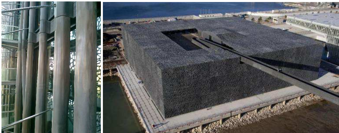
Figure 12: the MuCEM in Marseille [23-26]: 330 UHPFRC post-tensioned columns, 380 net cladding and roofing UHPFRC panels, two UHPFRC footbridges.
