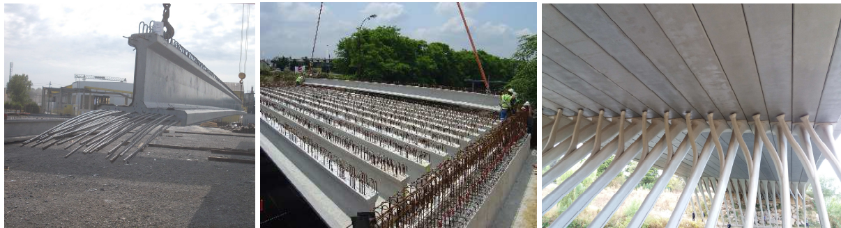
Figure 7: ITE® beams. Left) Just handled after precasting for Buthaumont Bridge [11]. Center) Being installed at Pinel Bridge, allowing safe deck completion from above [12]. Right) After completion, deck from below: Pont de la République in Montpellier [13]
