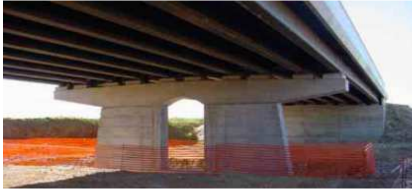
Figure 4: Bourg-lès-Valence UHPFRC bridge deck made of prestressed Pi-shaped beams.
