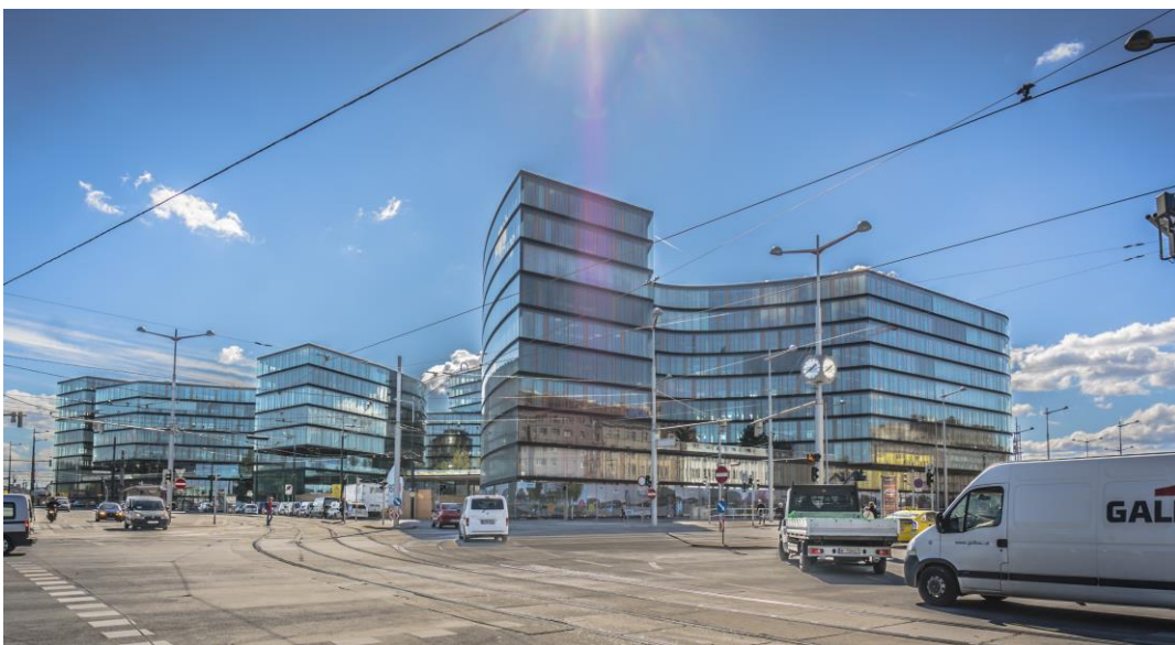
Figure 4: Central Train Station District office architecture (photo: M. Reisenleitner)
