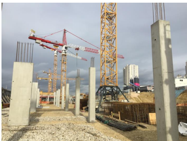
Figure I.9. Chapelle International Sogaris logistics hotel building site, 27 January 2016 Source: photo L. Dablanc
