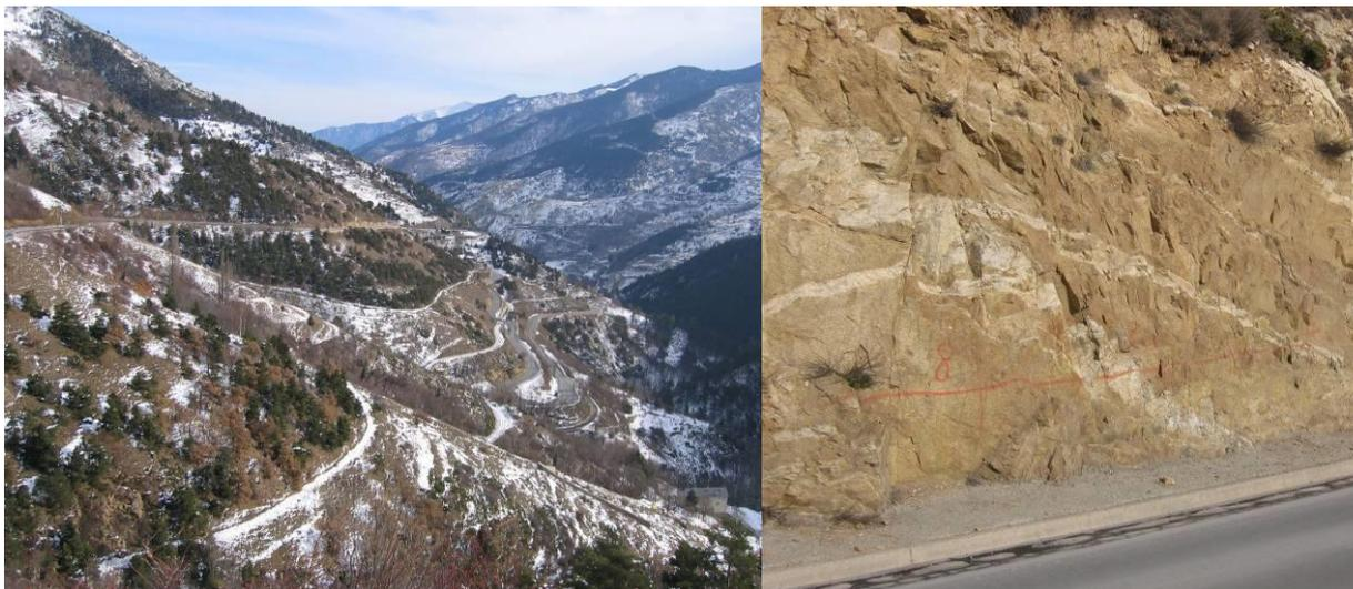
Fig. 1. Left: Panoramic view of the sector of Pallat, showing the existence of danger due to rock mass instability- Right: close-up of the fracture system at the road side outcrop, and measuring scanline.
