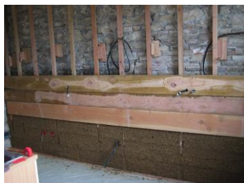
Figure 4: Banchage (200 – 500 kg/m 3 )
