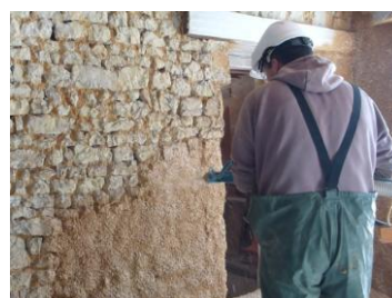
Figure 5: Projection (200 – 500 kg/m 3 )
