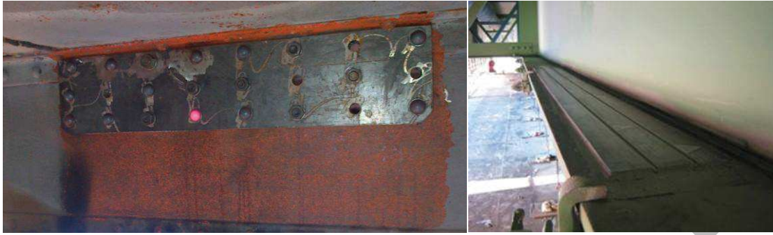
(a) (b) Figure 1: Pictures of repair solutions using (a) additional riveted steel plate, and (b) adhesively bonded CFRP plates (application on a construction site in France)
