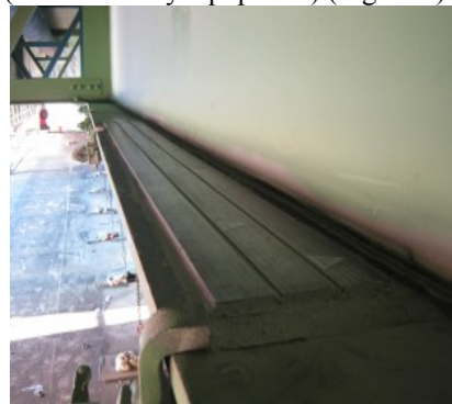
Figure 2. Adhesively bonded composite reinforcement
