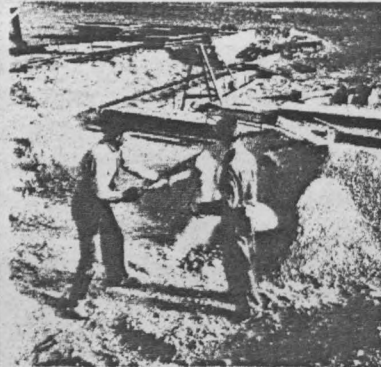
SOIL IS SIFTED through coarse mesh to remove stones and debris. Aggregates can range from fine sand up to large gravel but finer particles must predominate.
