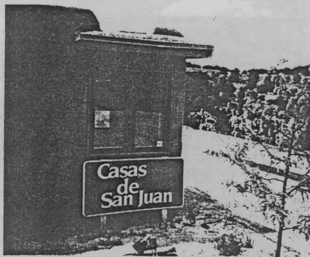
Don Woodman of Rammed Earth Contractors in Santa Fé stands before one of REC's recent rammed earth projects at Casas de San Juan, north of the city. Don and partner Richard Yates contracted for 500 linear feet of 12" thick wall in this house. Woodman has been a major force for rammed earth in the area and has given a fair amount of spare time to its promotion.
