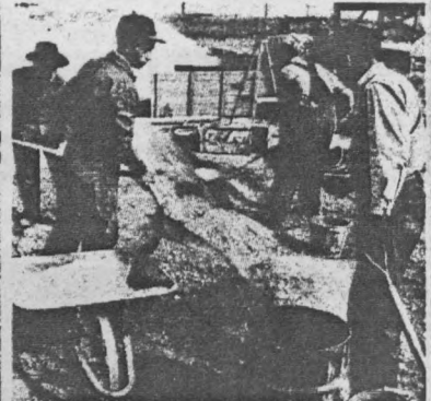
MIX IS DAMPENED by hand. Unlike adobe, terra pise is barely moistened. Soils with high clay content are unsuitable due to high shrinkage and high erosion of clay.
